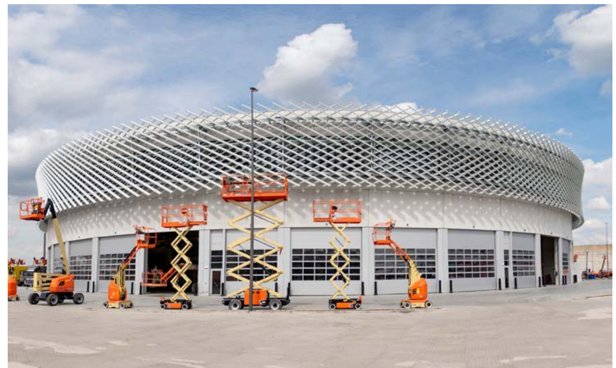
TVH Equipment in Waregem (BE); PRODUCT: MD Lamel, MD Flack; FIXTURES: project special; MATERIAL: Aluminium; FINISHES: Powder-coating RAL 7037; ARCHITECT: Demo Architecten, Izegem (BE)
