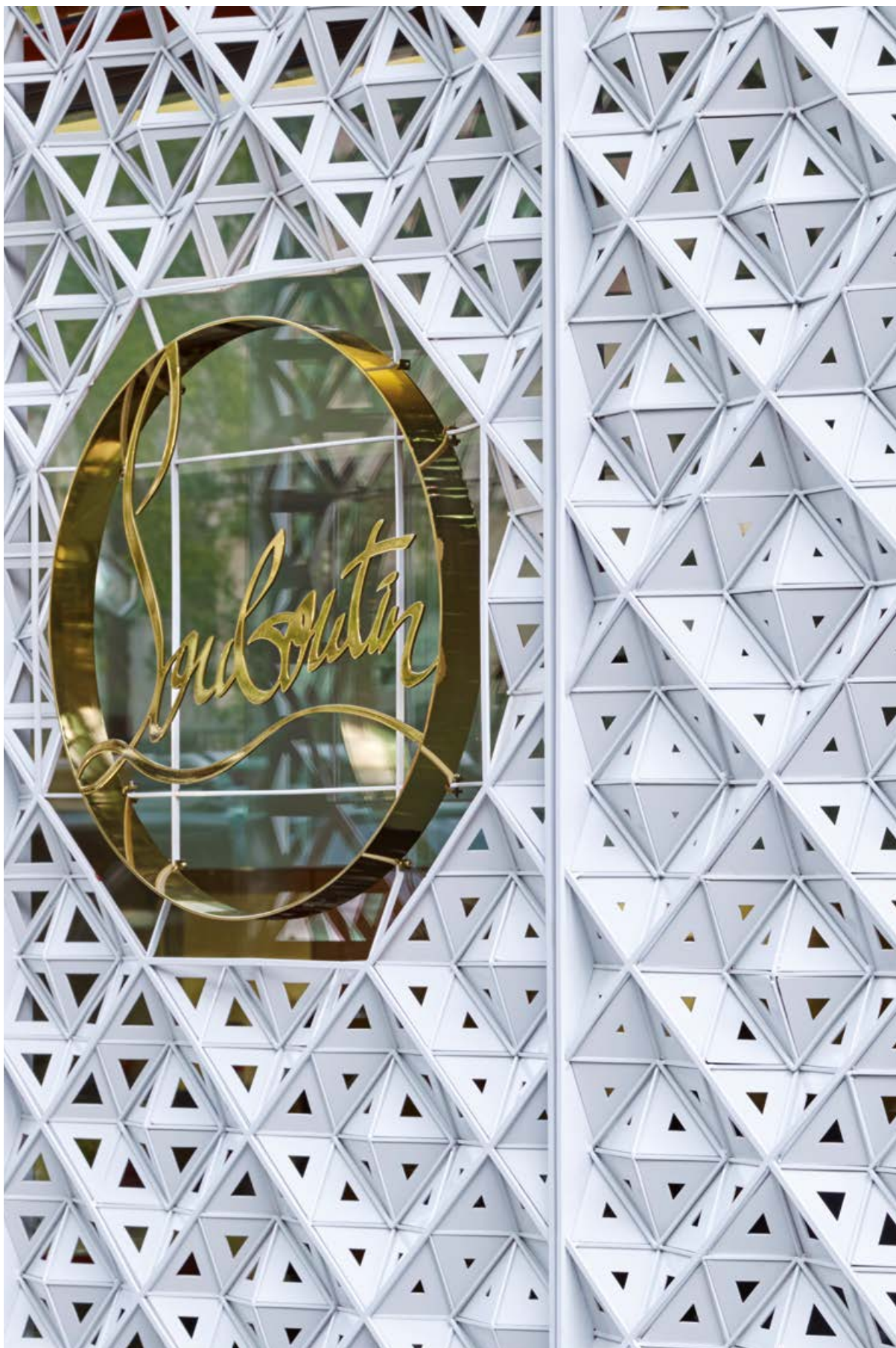
Shopfront Christian Louboutin on Madison Ave in New York; PRODUCT: MD Formatura and MD Shapes; FIXTURES: MD Resto; MATERIAL: Aluminium; FINISHES: powder coated in RAL 9001; ARCHITECT: 212box architects, New York
