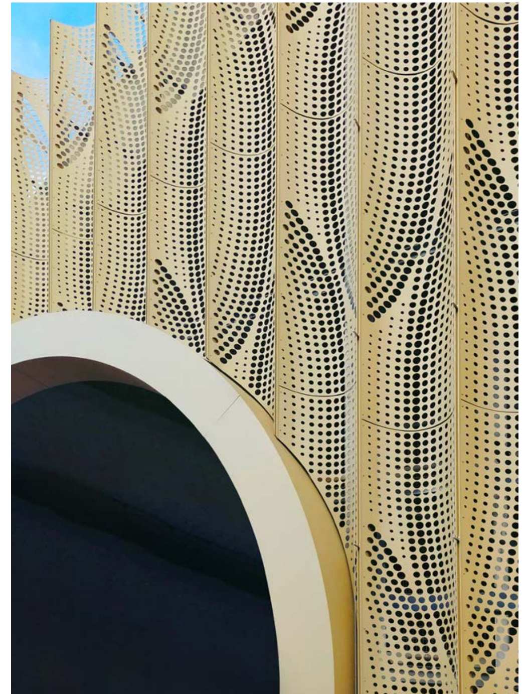
Parking Garage Hart van de Waalsprong in Nijmegen (NL); PRODUCT: MD Shapes with MD Designperforation; FIXTURES: MD Vertii; MATERIAL: Aluminium; FINISHES: Powder coated in metallic gold; ARCHITECT: korth tielens architecten, Amsterdam
