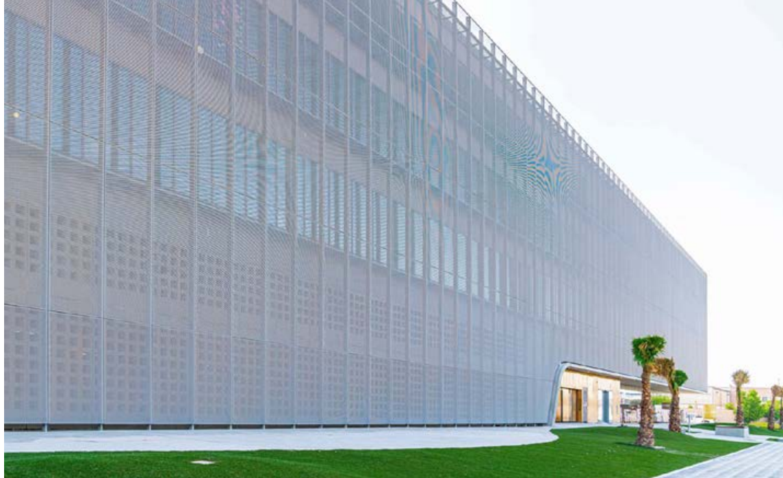
Raqtan Headquarters in Dammam (KSA); PRODUCT: MD Expanded Metal, MD Formatura (patio); FIXTURES: MD Resto; MATERIAL: Aluminium; FINISHES: Powder-coating in chrome; ARCHITECT: Rempt van der Donk, Rotterdam (NL)
