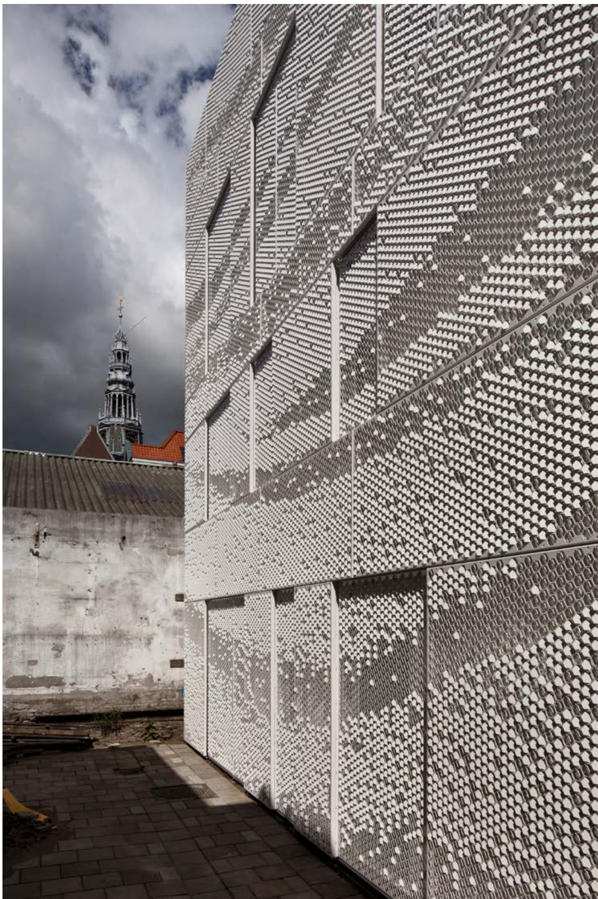
Residential Complex ‘Between the Sheets’ in Amsterdam (NL); PRODUCT: MD Formatura; FIXTURES: MD Resto; MATERIAL: Aluminium; FINISHES: powder coated; ARCHITECT: Abbink X Co, Amsterdam; ARTIST PATTERN: Chris Kabel
