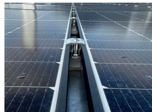
MidGrab module clamp can be used as Middle- and End-Clamp.
