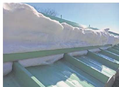
S-5!® ColorGard® mounted on S-5!® clamps with two set screws
